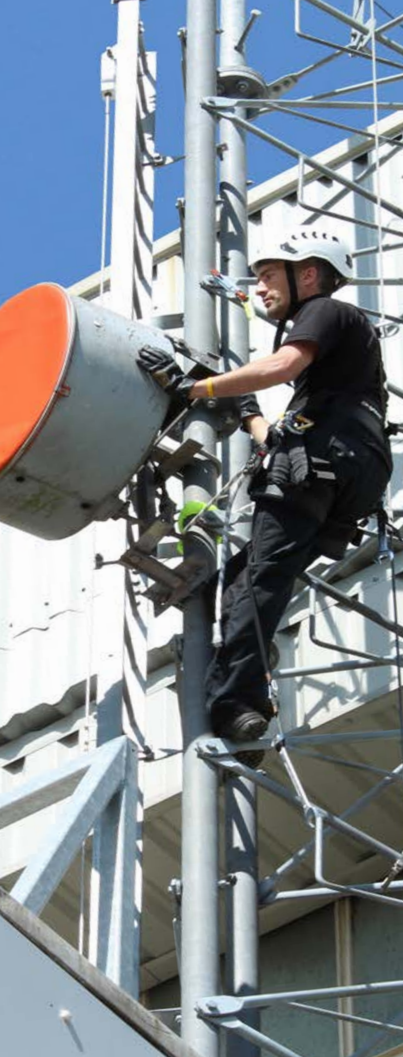
MATS Initial Basic Tower Climbing and Rescue - ARQIVA Gateway Approved
